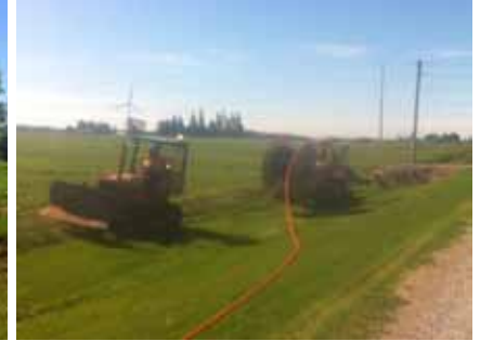
Pickards Construction crews working hard ploughing Fibre on Parr Line near Centennial Road.
